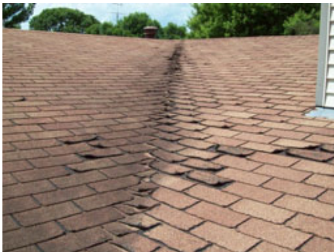
Valley, south west side
